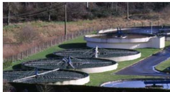
Station d'épuration © Marc Rappilliard
