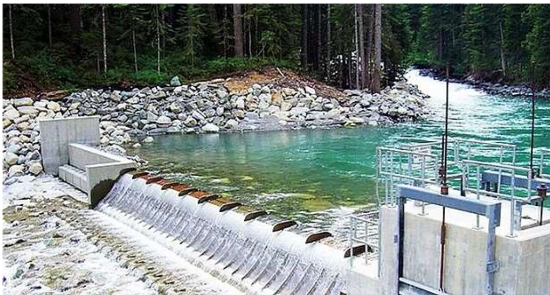
Small hydropower plant in Republika Srpska, Bosnia and Hercegovina
