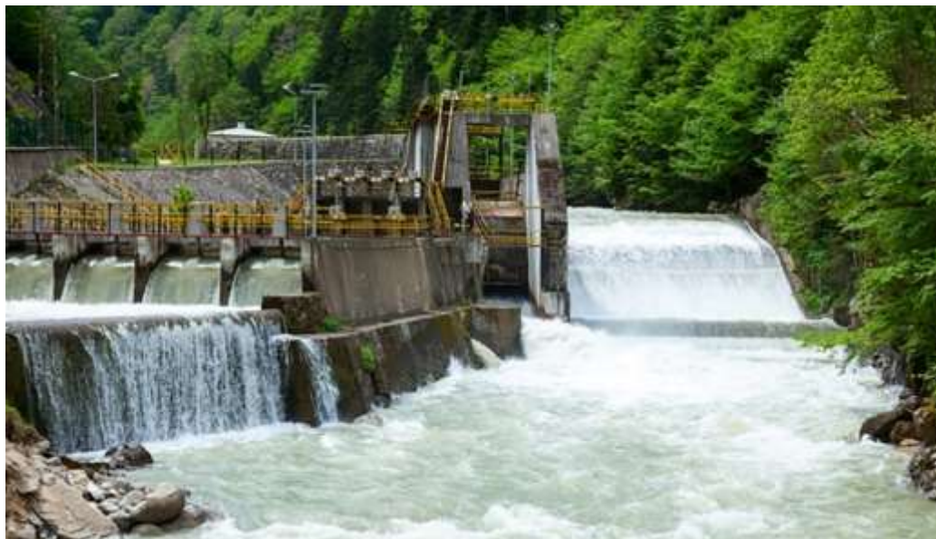
Small hydropower plant
